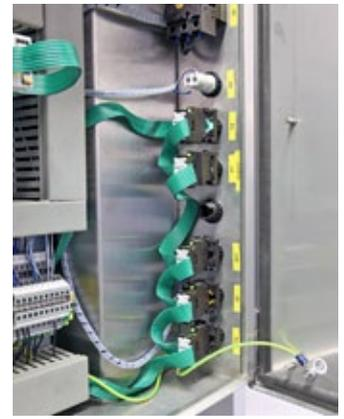
The wiring of the operating elements can also be implemented easily via SmartWire-DT, with which a green light on every slave is used to indicate operational readiness
